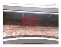
There are large gaps over 1/4" in size adjacent the beam. These gaps allow insects and rodents to enter the attic. Covering the gaps with screening, a strip of wood and/or caulking is recommended.
