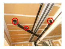
The installation of a furnace vent thimble is recommended to prevent flames from spreading to the structure.
