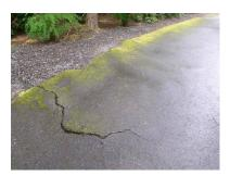
Large cracks were observed in the asphalt surface of the driveway. Cracks can be sealed to minimize moisture entry, vegetation establishment and further settlement of the asphalt. Minor cracks are common and do not affect the serviceability of the asphalt.
