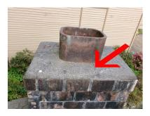
The top of the masonry chimney does not have a spark arrestor/rain cap. The installation of a spark arrestor/rain cap is recommended as a safety upgrade and to prevent moisture damage to the inside of the chimney and fireplace. An additional benefit of a rain cap is that it will keep birds and rodents from entering the house when the damper is left open.
