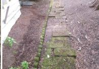
The walking surface was not even and trip hazards were present. We recommend all walking surfaces be maintained free of trip hazards.
