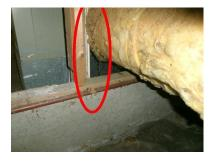
Scrap-wood and other cellulose debris was observed on the crawl floor. This wood debris creates conducive conditions for wood boring insects. The removal of all cellulose debris is recommended.
