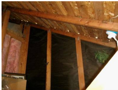
Openings observed from within attic
