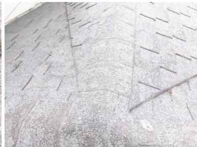
Heavy loss at ridge observed
