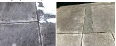
The wooden dividers separating the concrete walkway sections have deteriorated to a point where the gaps are a trip hazard. Replacement with mortar is recommended.
