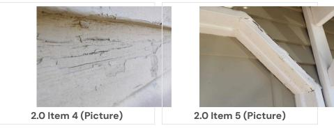
(2) Wood rot was found on the lap siding and trim pieces of the home. I would recommend having a contractor to further evaluate and remove any rotten wood pieces and replace with prepped and painted pieces.
