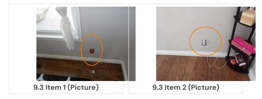
(2) The 220 outlet for the dryer is loose and should be securely fastened to the wall. Any movement in receptacles like this can lead to loose or worn out wires and could become a fire hazard.
