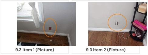
(2) The 220 outlet for the dryer is loose and should be securely fastened to the wall. Any movement in receptacles like this can lead to loose or worn out wires and could become a fire hazard.
