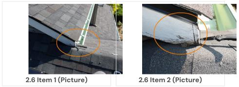
(2) The paint on the soffit and fascia is failing. I recommend that a professional painting company evaluate, prep and re-paint in the near future.
