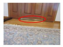
The garage side door has a thin panel at the bottom which can easily be kicked in. Replacing or reinforcing the door is recommended to enhance your personal security.
