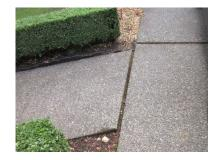
The walking surface was not even and trip hazards were present. We recommend all walking surfaces be maintained free of trip hazards.
