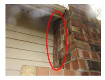
The kick out flashing at the roof edge to wall intersection above the gutter is too small. This will allow water to enter the wall behind the siding. The installation of a larger kick-out flashing is recommended.
