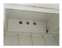
There are openings at the intersection between the overhang and the brick facade through which birds and rodents can enter into the attic. These openings should be covered with wood, wire mesh or filled with aerosol foam.
