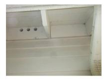
There is a damaged vent screen on the front of the house. The vent screen should be repaired to prevent insect, bird and rodent entry.
