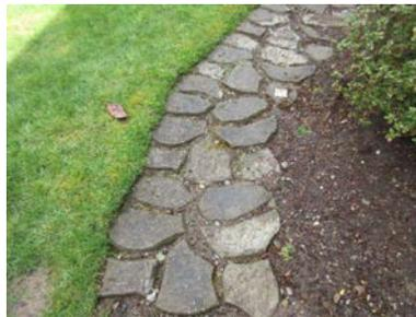
The walking surface was not even and trip hazards were present. We recommend all walking surfaces be maintained free of trip hazards.
