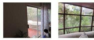
The lower window glass is not labeled as tempered safety glass. The existing glass is nonconforming by current building standards and would be hazardous if broken. The installation of safety glass is recommended as a safety upgrade for all windows less than 18" from the walking surface.
