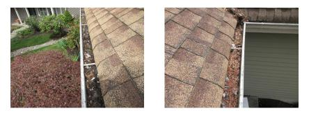
Downspouts draining directly onto the asphalt shingle surface causes excessive wear of the roofing material. Downspout extensions to the lower gutters should be installed to prevent excessive wear and tear of the roofing.
