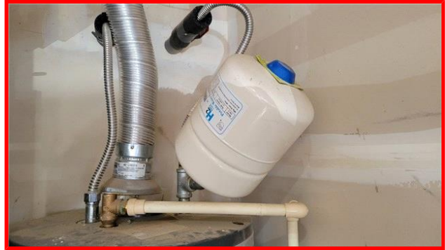
Failed Expansion Tank
