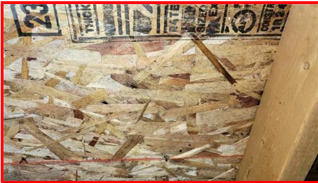
Suspect Mold on Sheathing
