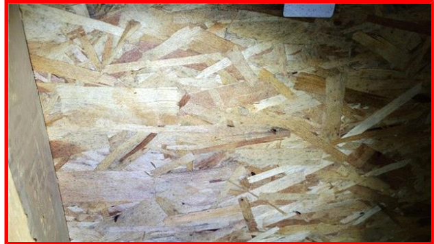
Suspect Mold on Sheathing
