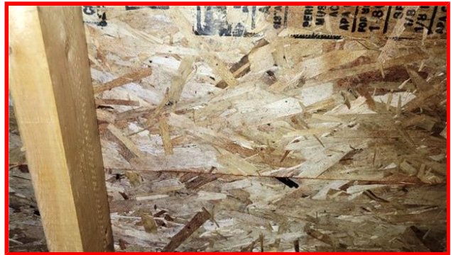
Suspect Mold on Sheathing
