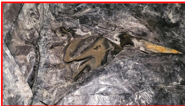
Standing Water in Crawl Space Near Access
