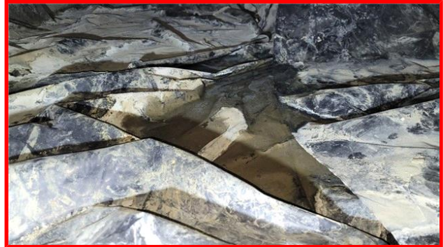
Standing Water in Crawl Space Below Bathroom
