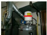
RECIRCULATING PUMP The recirculating pump above the water heater pumps hot water through a loop that
