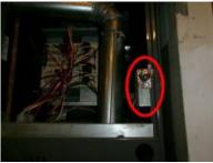
AIR FILTER The air filter is located in the return air plenum adjacent to the furnace. The air filter should be cleaned or replaced at least 2-3 times during the heating season.
