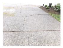
One or more of the wooden dividers separating the concrete driveway sections were infested by wood destroying organisms and have deteriorated to a point where they are becoming a trip hazard. Replacement with mortar is recommended.
