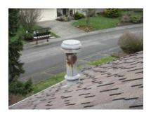
The storm collar is not sealed. This is allowing leakage to occur. Sealing the storm collar is recommended.
