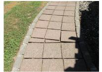
The minor settlement of the patio blocks and the gaps separating the patio stones are a trip hazard. We recommend all walking surfaces be maintained free of trip hazards.
