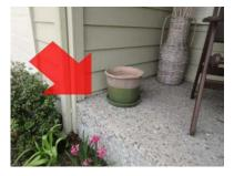
There are openings adjacent pipe and wire penetrations at the exterior wall through which rodents and other pests can enter into the structure. These openings should be covered with wood, wire mesh or filled with aerosol foam.
