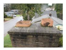
Mortar was missing or deteriorated in numerous areas around the chimney. This has led to accelerated deterioration of the brick masonry. Damaged areas can be repaired by filling in cutout or defective mortar joints with fresh mortar. (Tuck pointing)
