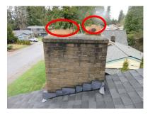
The chimney crown is cracked and deteriorated. The mortar chimney crown prevents water from entering and damaging the masonry. Repairing or replacing the chimney crown will extend the service life of the chimney.
