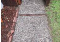
There is no handrail along the stairs. This is a hazard. The installation of a handrail along the stairs is recommended.
