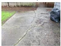
The wooden dividers separating the concrete walkway sections have deteriorated to a point where the gaps are a trip hazard. Replacement with mortar is recommended.
