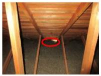
VENTILATION Flexible plastic duct is used to direct air from the vent fans to the exterior. This type of material is unreliable. Replacing the plastic duct with 4" smooth-wall sheet metal duct is recommended.
