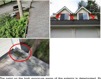
The paint on the high exposure areas of the exterior is deteriorated. Paint protects the wood from cupping, checking, warping and rot. Repainting the exposed areas is recommended.
