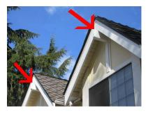
There are openings at the intersection between the vent blocks and the brick cladding through which birds and rodents can enter into the attic. These openings should be covered with wood, wire mesh or filled with aerosol
