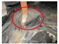
Cellulose forms were left in place on the pier footings. This cellulose is conducive to the infestation of various wood destroying organisms. The removal of the cellulose is recommended.
