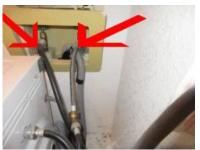
The visible portions of the dryer vent are properly installed and in serviceable condition. Dryer ducts should be cleaned annually as part of routine home maintenance. A dryer duct that is clogged with lint is a fire hazard.
