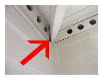
The beams that stick out beyond the drip edge of the roof are vulnerable to rot damage. They should be covered with a metal cap flashing or cut off flush with the edge of the overhang.
