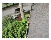
Downspouts draining directly onto the asphalt shingle surface causes excessive wear of the roofing material. Downspout extensions to the lower gutters should be installed to prevent excessive wear and tear of the roofing.
