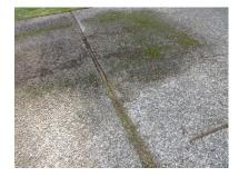
The wooden divider separating the concrete driveway sections has deteriorated to a point where it is a trip hazard. Replacement with mortar is recommended.
