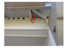
The beams that stick out beyond the drip edge of the roof are vulnerable to rot damage. They should be covered with a metal cap flashing or cut off flush with the edge of the overhang.
