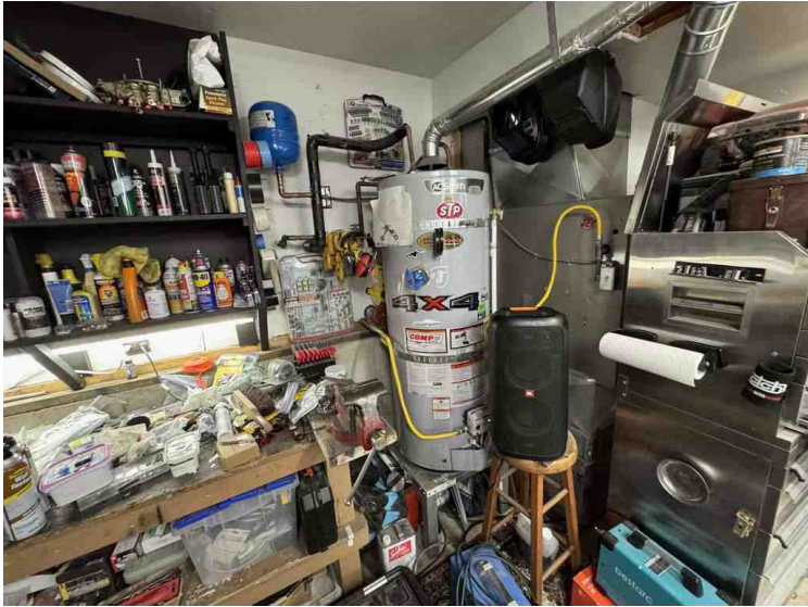
Subjects Hot Water Tank with Double Seismic Straps
